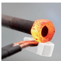
Releasing of rusted bolts
